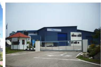
Plant expansion, Bentong
